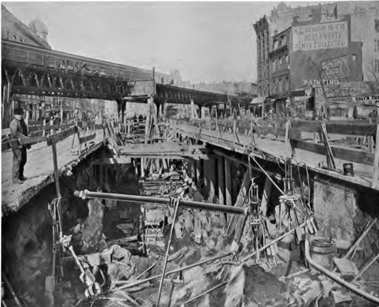
SUPPORTING ELEVATED RAILROAD BY EXTENSION GIRDER—64TH STREET AND BROADWAY
